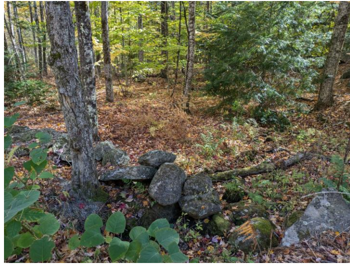
View from culvert south along stream
